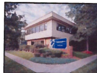
Mulberry Office 401 W. Mulberry Street Fort Collins, CO 80521
