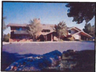
Loveland Office 1401 W. 29th Street Loveland, CO 80538
