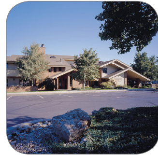
Loveland Office 1401 W. 29th Street Loveland, CO 80538 970.663.0700
