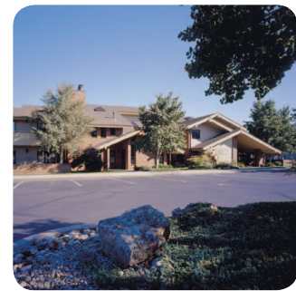
Loveland Office 1401 W. 29th Street Loveland, CO 80538 970.663.0700
