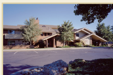
Loveland Office 1401 W. 29th Street Loveland, CO 80537 (970) 663-0700
